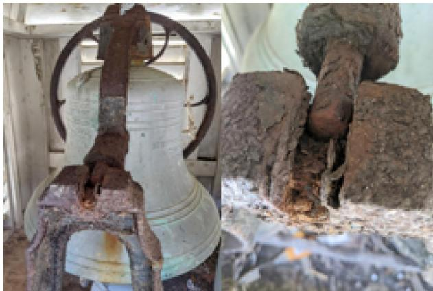
Bob Johnson secured a tow behind man lift and oversaw the repair, which went very well. After the bell was secured on the new stands, all other parts including the bell, bearings, and wheel were cleaned and lubricated. After cleaning, all existing parts, except for the bell, were painted. A new pull cord was also installed.
